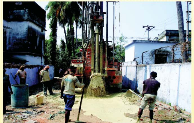
Deep Bore Well work in progress
